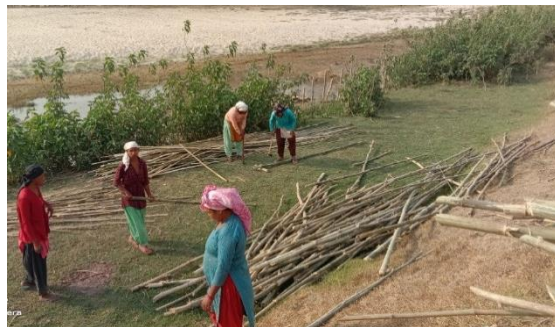
Women working on bio-engineering works-Photo KMJS for USAID
